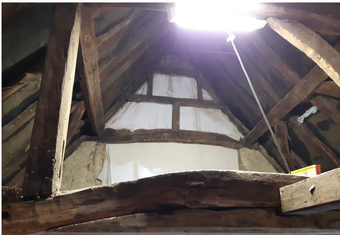
Image – Roof structure, Old Bakehouse, N. Crawley
